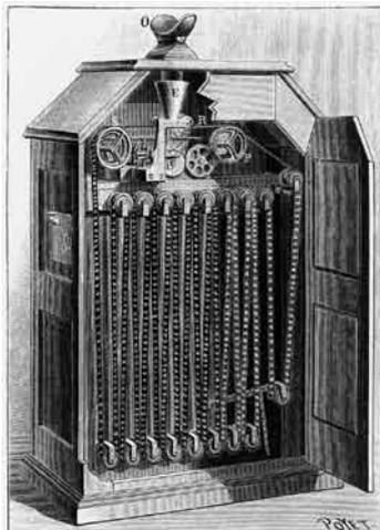
He produced the *kinetoscope*, which was an early version of the film projector.
